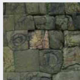
24. Stone Retaining wall
