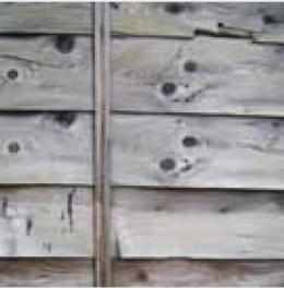
6. Wood cladding (over earth walls)
