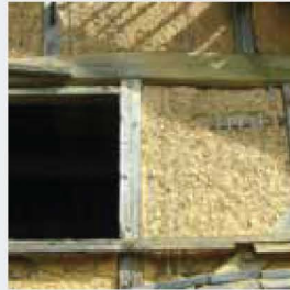
8. Plaster and wood structure (over earth walls)
