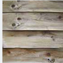
9. Board wood walls
