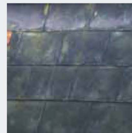
15. Copper plate roof
